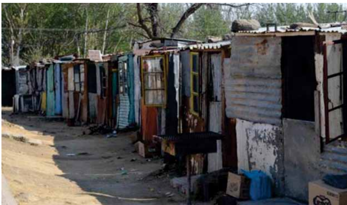
Some of the shacks surrounding the bus shelter area, Mohale's Hoek, Lesotho.
